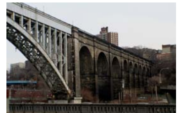
High Bridge with steel arches C.A. 1990
